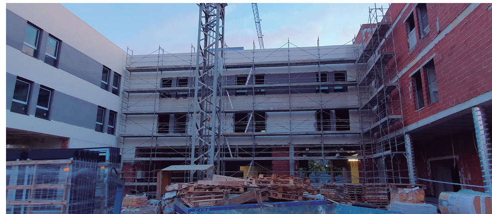
Valencia project during its construction
