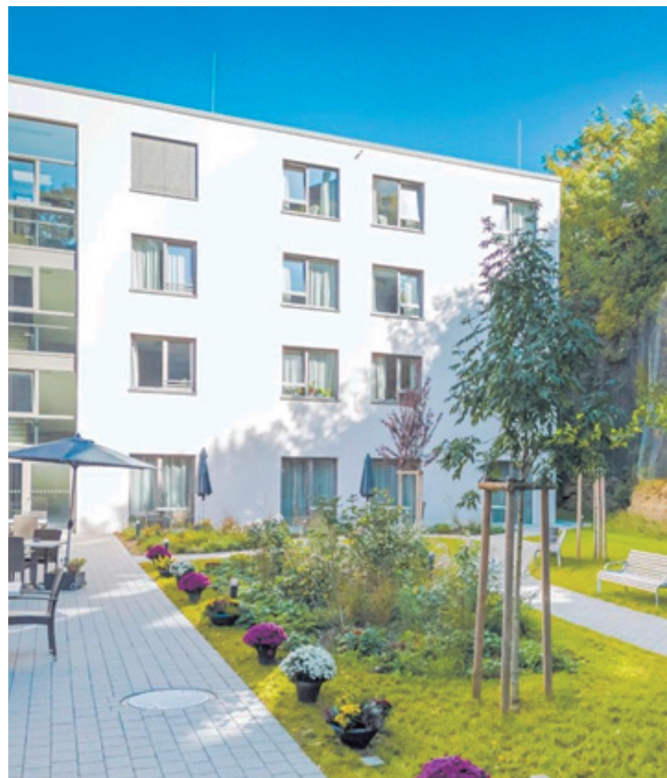
Erdmannhausen Nursing Home in Germany
