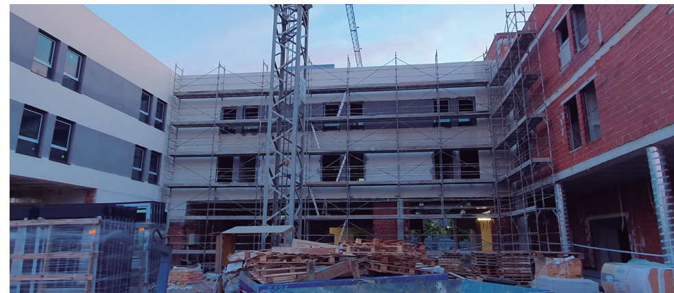
Valencia project during its construction
